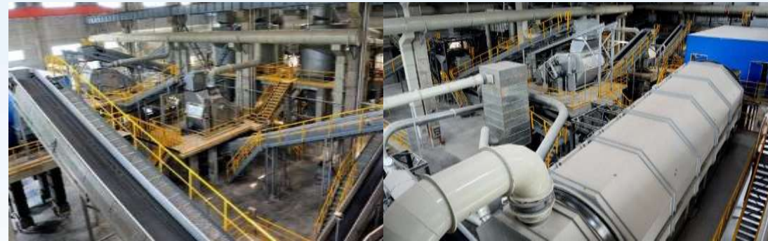
• Municipal Waste Treatment Plant
