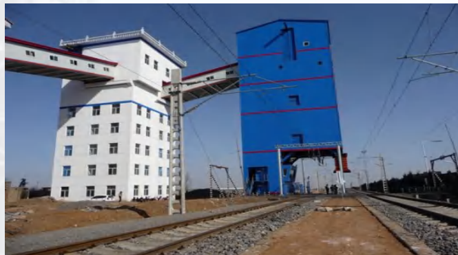
Train/Truck Loading Terminal
